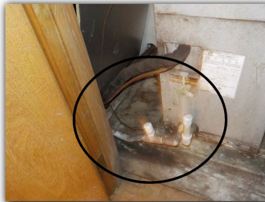
HVAC closet on second floor
