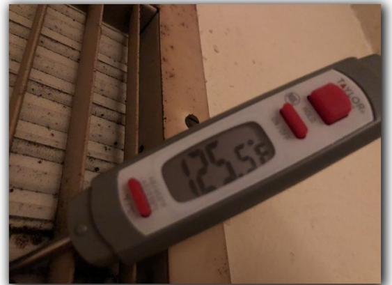
Supply air / differential
