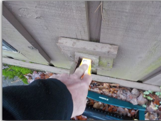
Missing GFCI protection on exterior of home
