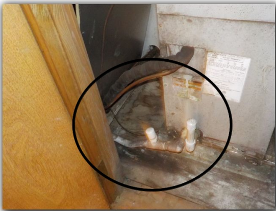
HVAC closet on second floor
