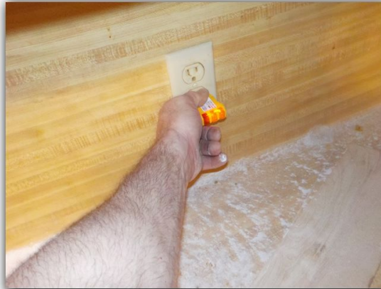
Missing GFCI protection in kitchen area
