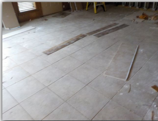
Views of ceilings and floors
