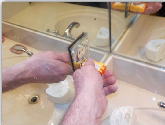
Master bathroom Missing GFCI protection in bathrooms
