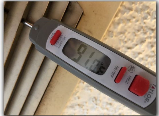
Supply air / differential
