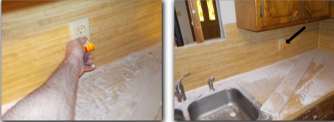
Missing GFCI protection in kitchen area
