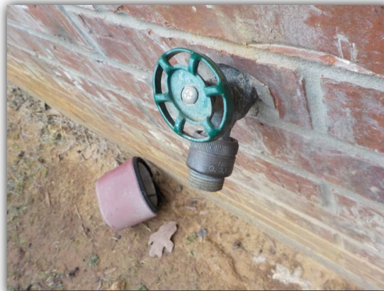
Back flow preventer in place at time of inspection.
