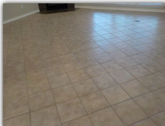
Views of ceilings and floors
